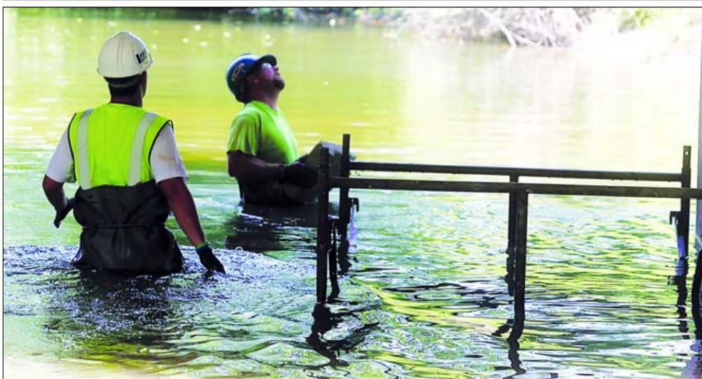
**ABOVE:** Rick Hoer Jr., left, and Chris Johnstone from Lakeside Construction had the coolest job at the site of a bridge rehab project on Route 565 in Frankford Tuesday afternoon. The pair built scaffolding under the bridge so a crane can be hooked to old beams to lift them out.
